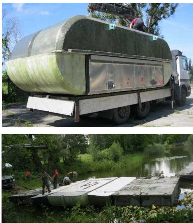
Fig. 6. Segment transport and construction of the crossing in combination with PP-64 segments
