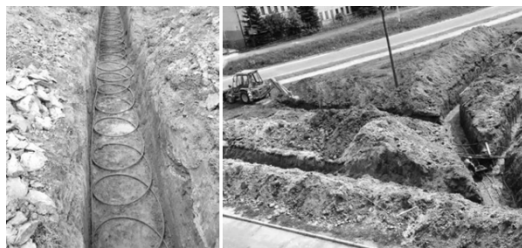
Fig. 1. Ground heat exchanger
