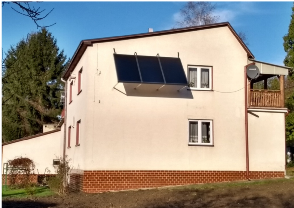
Fig. 5. Solar collectors on the facade, Błazowa. Source: own study
