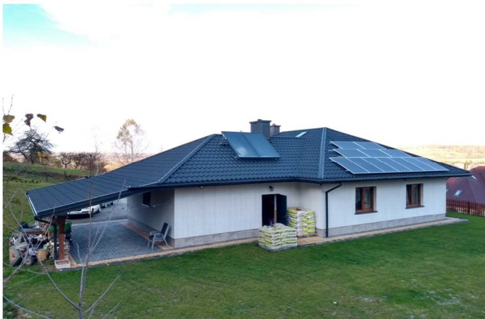
Fig. 6. Solar panels and collectors, Błazowa Dolna. Source: own study
