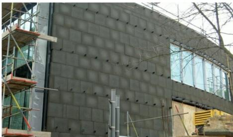
Fig. 8. Foam glass insulation
