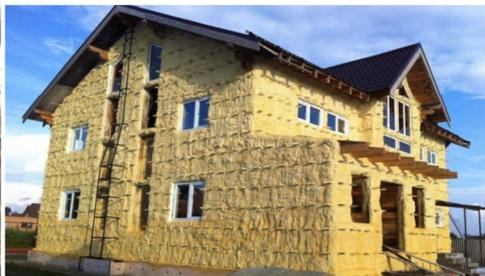
Fig. 9. Polyurethane foam insulation
