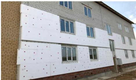
Fig. 6. Basalt mineral wool insulation
