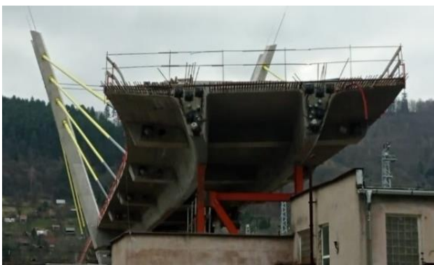
Fig. 3. Box girder bridge: extradosed bridge in Zilina
